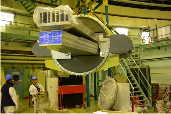
Fig. 11.1: The exchange of beam-tubes such as the H1-H2 shown here is part of the continuous upgrade of key reactor components.
