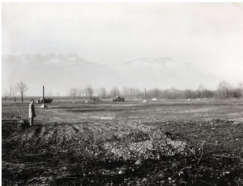
Fig. 7.1: View of the site where the ILL will be built.
