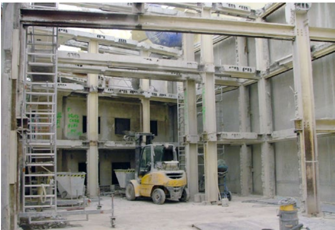
Fig. 11.6: Demolition and removal of internal structures at the top level of the ILL building to reduce inertia in case of a seismic event.
