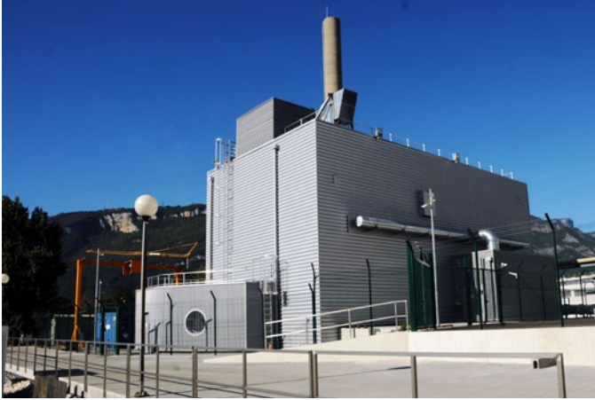
Fig. 11.7: The new highly reinforced building hosting both the heavy water treatment facility and, on the roof, the emergency control room PCS3.
