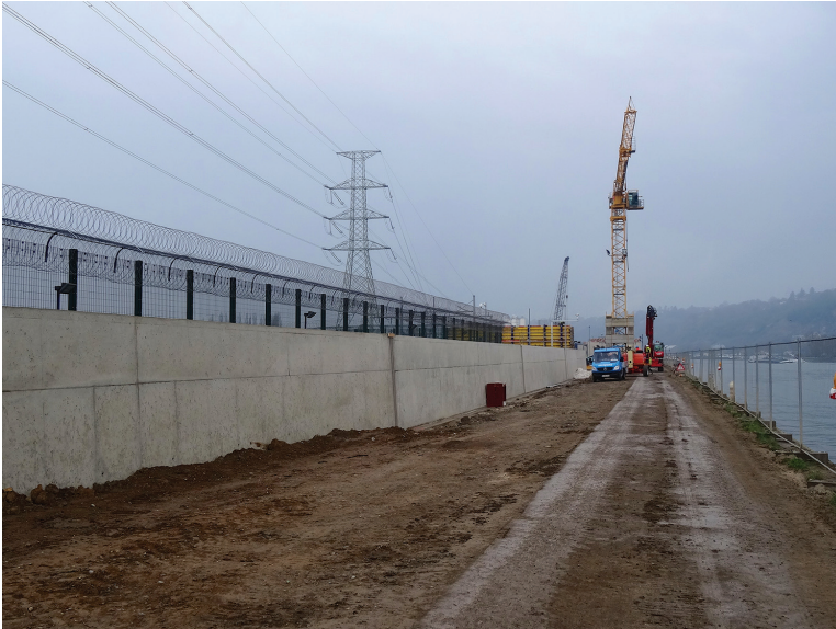
Figure 37.2. Peripheral protection of the Tihange site. Tihange nuclear power plant.
