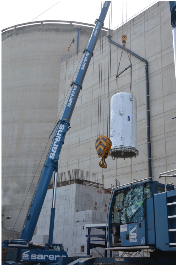
Figure 37.4. Installing the filter in Tihange Unit 3. Tihange nuclear power plant.
